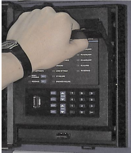
Figure 2-6: ROTATE HANDLE TO STOP POSITION
